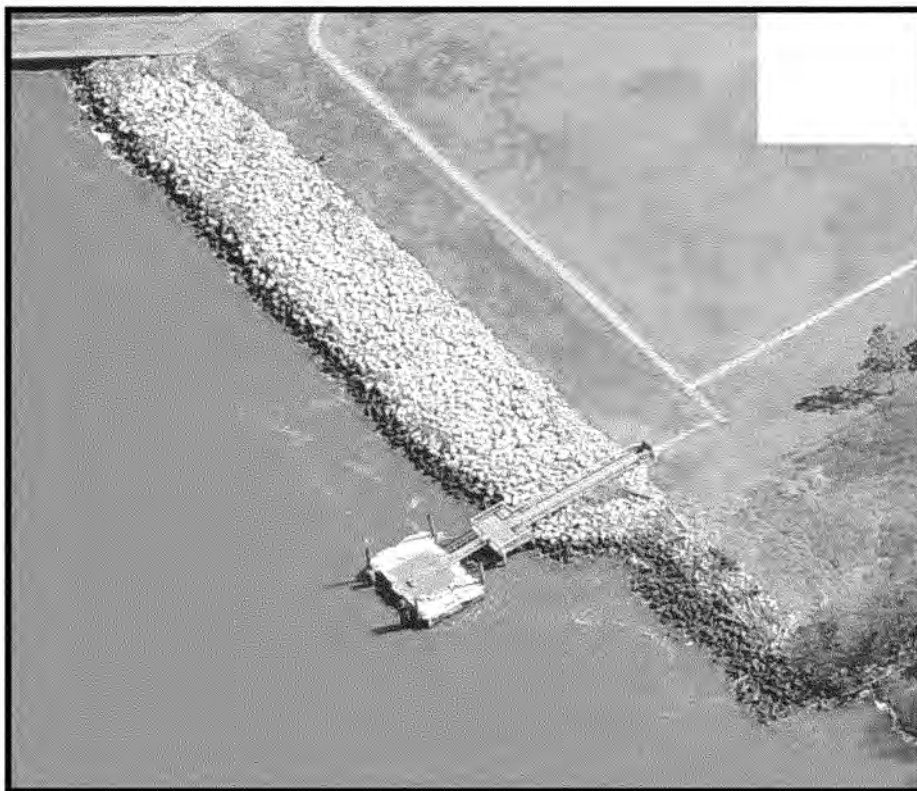
Figure 5-55. Upstream bank protection at Old Fort Jackson.
