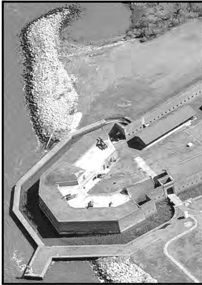
Figure 5-54. Aerial view of Old Fort Jackson.
