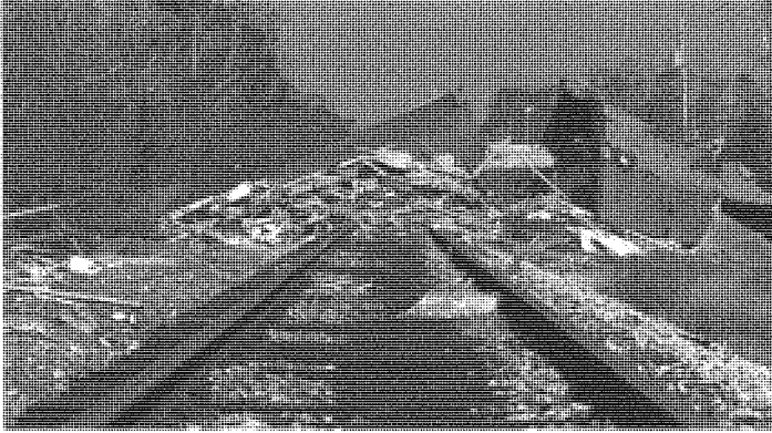
Figure ES-4. The CSX Railway parallels the coast and its embankment acted as a low levee-like storm surge barrier in some areas.
