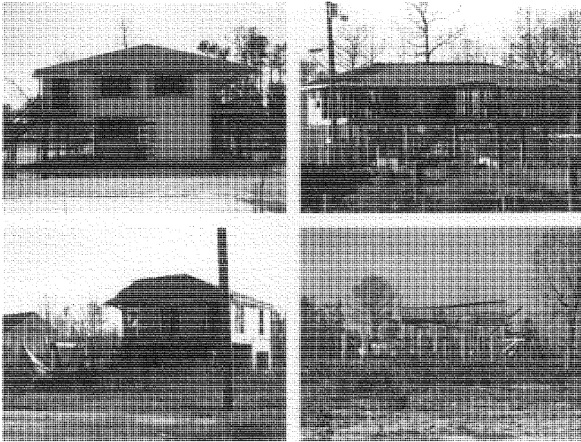
Figures 10, 11, 12 and 13. Damages to Elevated Structures
