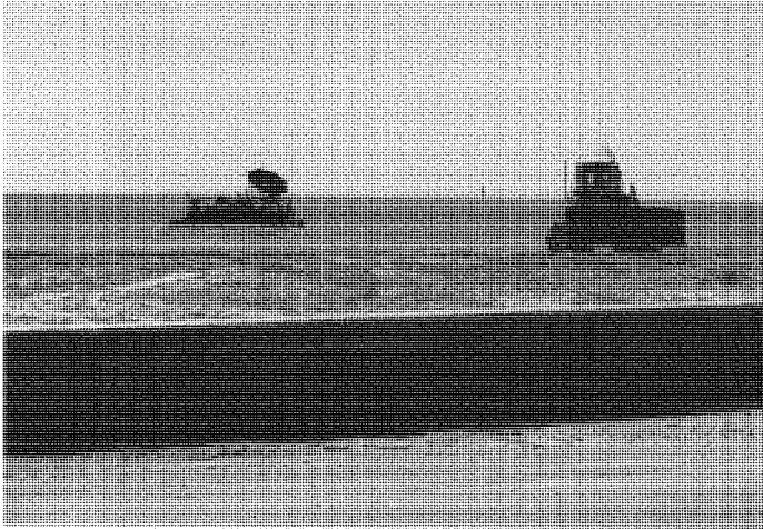
Figure 2.1.3-1. Photo of existing beach-front roadway and sea wall in Hancock County, June 2006. Equipment in the background is moving sand from the area just off-shore back onto the beach after being eroded by Hurricane Katrina.
