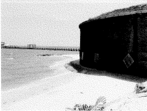
12 13 Figure 3.1.2.11-3. Photo of erosion on north side of Fort Massachusetts showing 14 relationship to encroaching waters to the structure. Note the small jetty that has 15 created severe scour at the down-current end.
