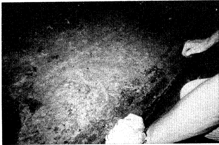
Inside Gate, Web Corrosion
