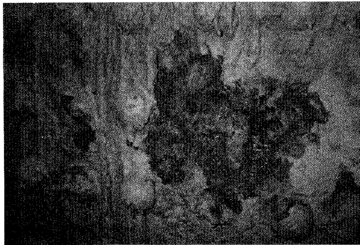
Inside Gate, Rivet Heads Protective Coating Gone and Heads Rusting Away
