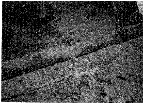
Inside Gate, Web Stiffener Angle Corroded Thru
