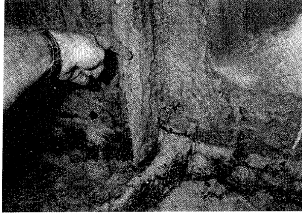
Inside Gate, General Corrosion
