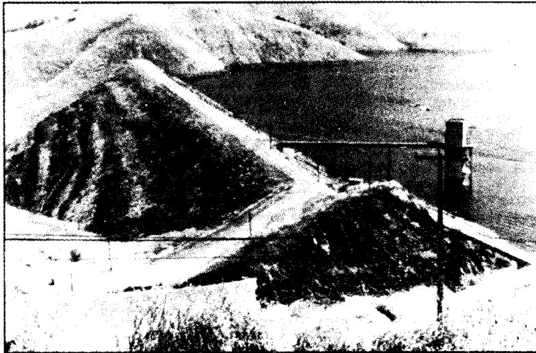
Terminus Dam and Lake Kaweah. Constructed in 1962 with an initial capacity of 150,000 acre-feet, it provides flood control and irrigation water supply storage, recreation, and hydropower benefits.
