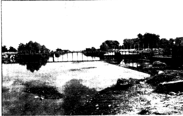
McKays Point flow division weir. Structure evenly divides flows from the Kaweah River into the St. Johns and Kaweah Rivers up to flows of 5,500 cfs.
