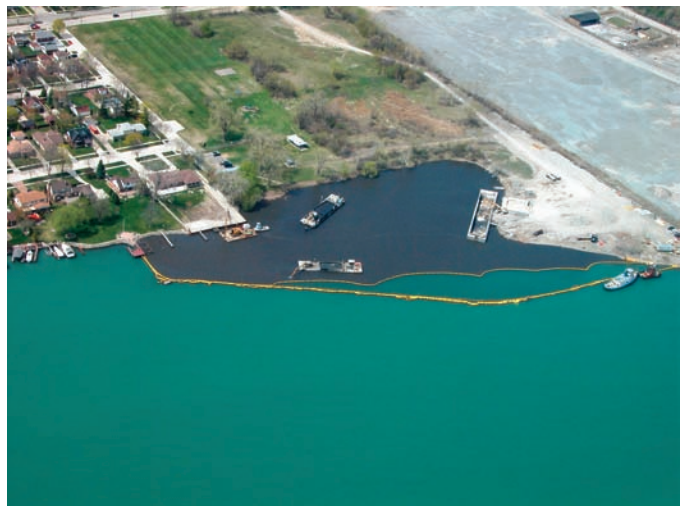
While EPA and the Michigan Department of Environmental Quality dredged the Black Lagoon, yellow silt barriers kept contaminated sediments from spreading in the Detroit River.
